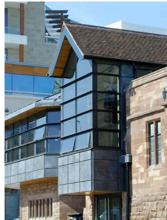
The Entrance Facade - St Martins Arts Cafe
